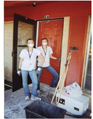
Ready to demolish!
